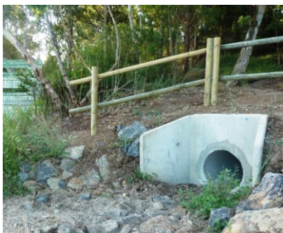
The storm water outlet into the north lake
